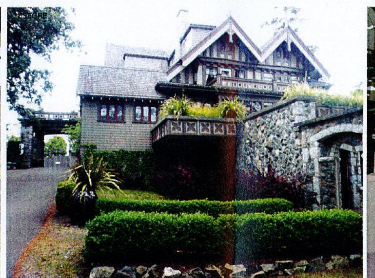
G4 EXISTING VIEW SHOWING EXISTING WINDOWS TO BE REPLACED.
