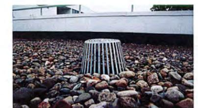
AREA DRAIN ON SLAB NOTE AGGREGATE ROCK SIZED TO BE LARGER THAN HOLES IN DRAIN COVER
