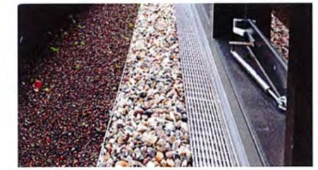
EXAMPLE OF MULTIPLE AGGREGATE SURFACE TYPES
