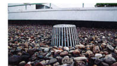
AREA DRAIN ON SLAB NOTE AGGREGATE ROCK SIZED TO BE LARGER THAN HOLES IN DRAIN COVER
