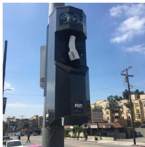
Example of an EV charging station mounted on a public utility pole in Los Angeles. Photo credit: Barry Lank
