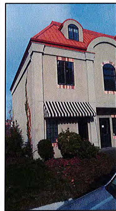
Existing Building: South East corner
