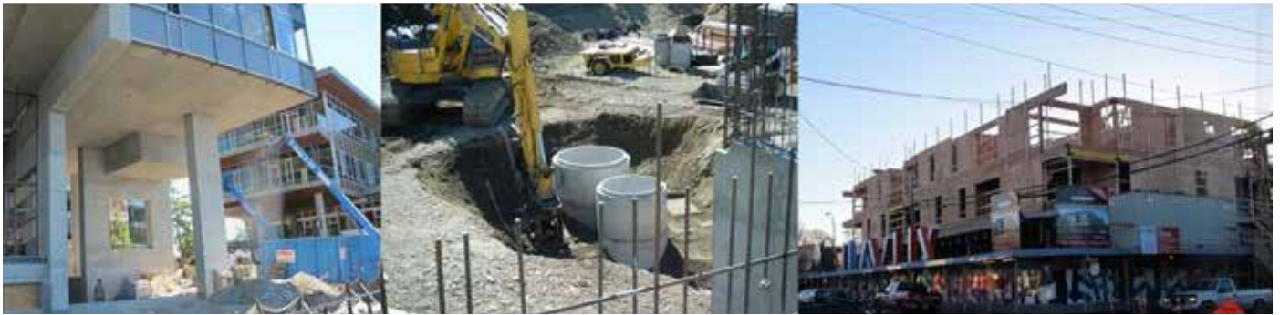
5. Pollution management protocols (including sedimentation and oil-removal), as well as recycling programs should be followed during demolition, excavation and construction of the project.
