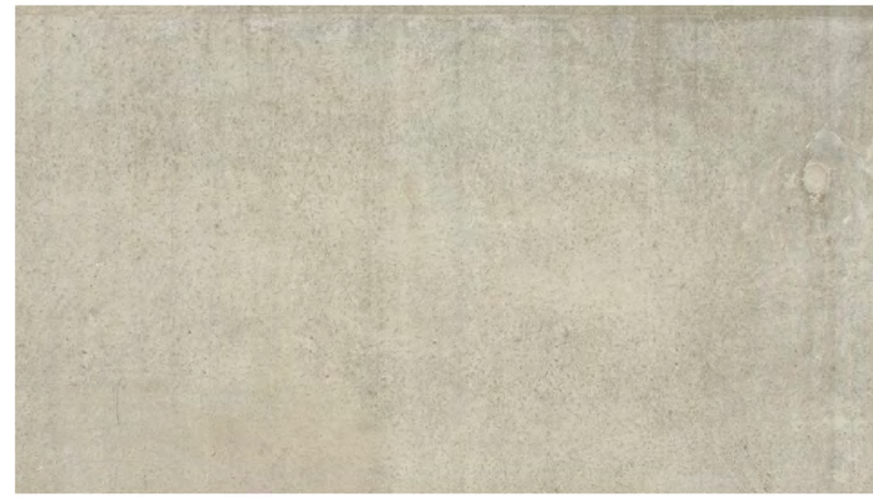
4 Board Form Concrete Base
