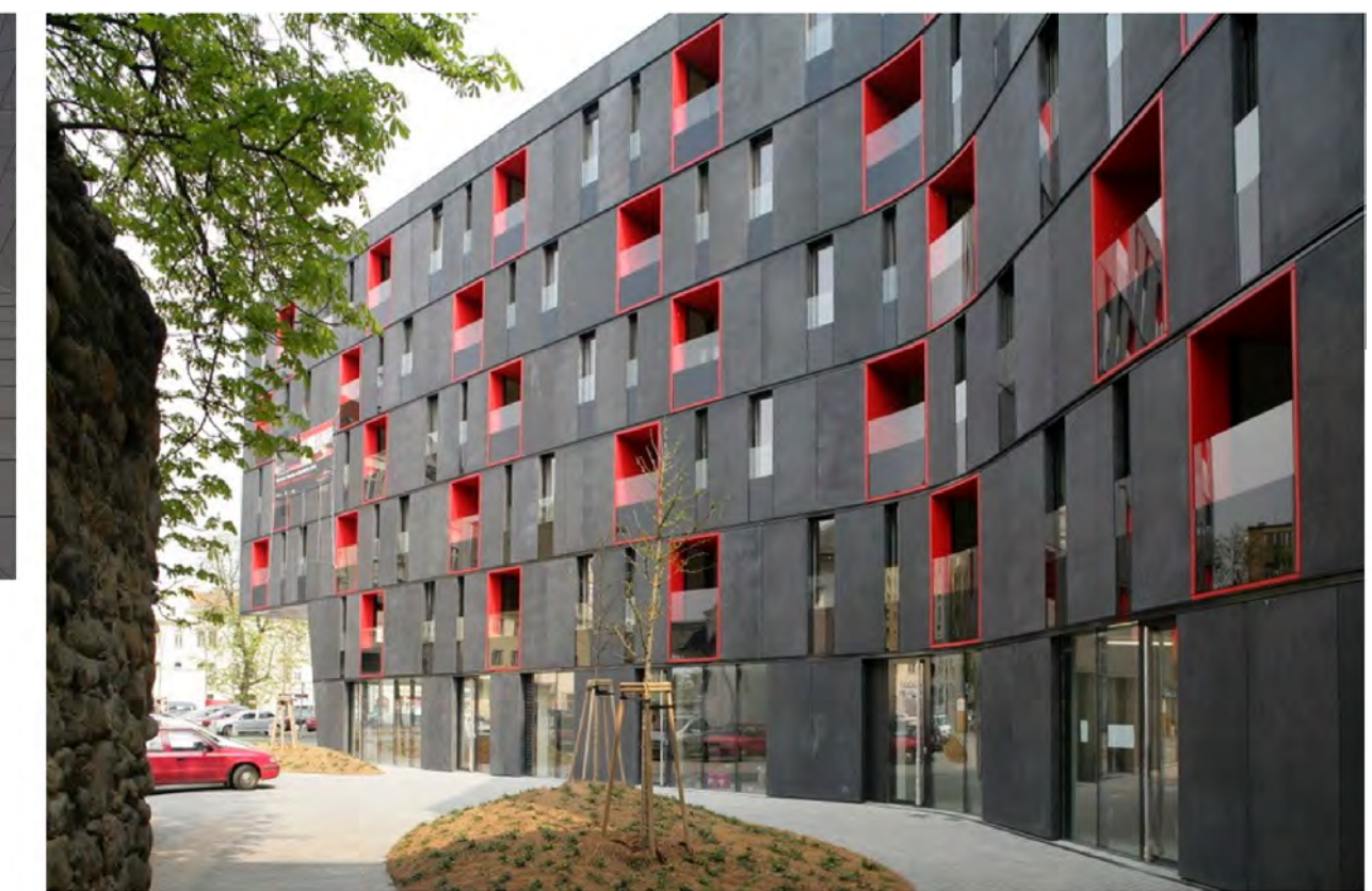
Ostrava City Gate by Kuba & Pilaf Architekti
