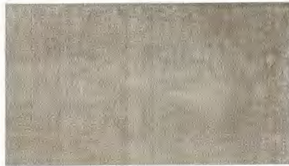
Board Form Concrete Base
