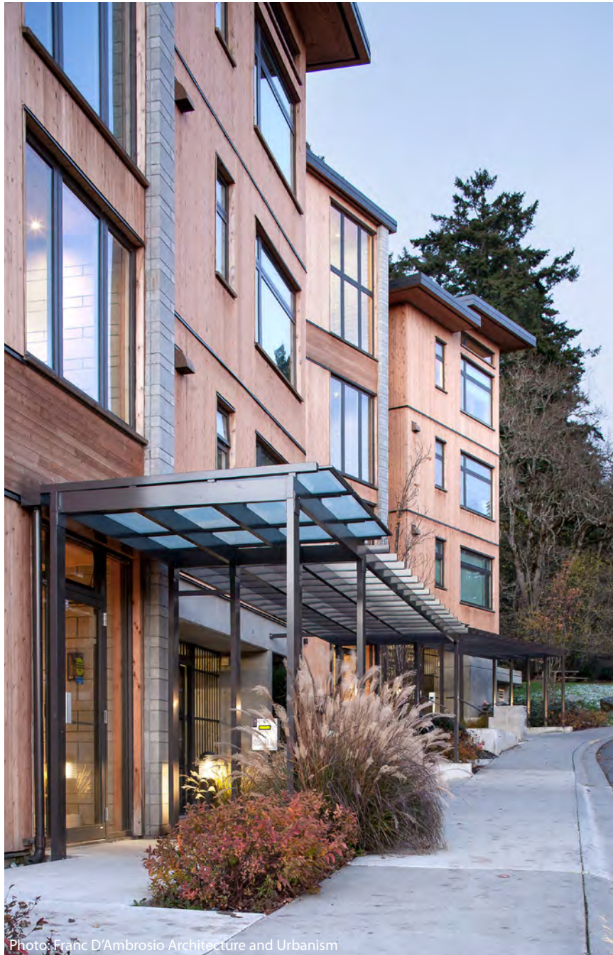
Photo: Franc D'Ambrosio Architecture and Urbanism
