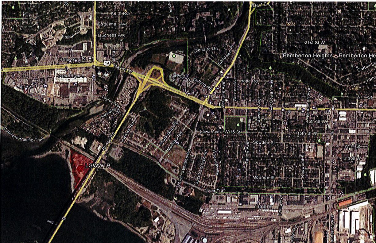
Figure 1: Lions Gate Wastewater Treatment Plant
