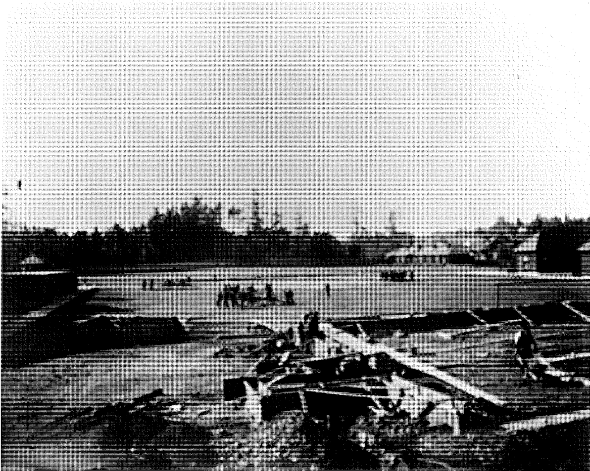
Work Point, looking west over the construction of the "Works Office" at Work Point Barracks circa 1893. In the background are the Royal Marine Artillery with their muzzle-loader carriage guns in the Parade Square and the Enlisted Men's Barracks to the far right. [Young Collection, Esquimalt Archives 994.4.7]
