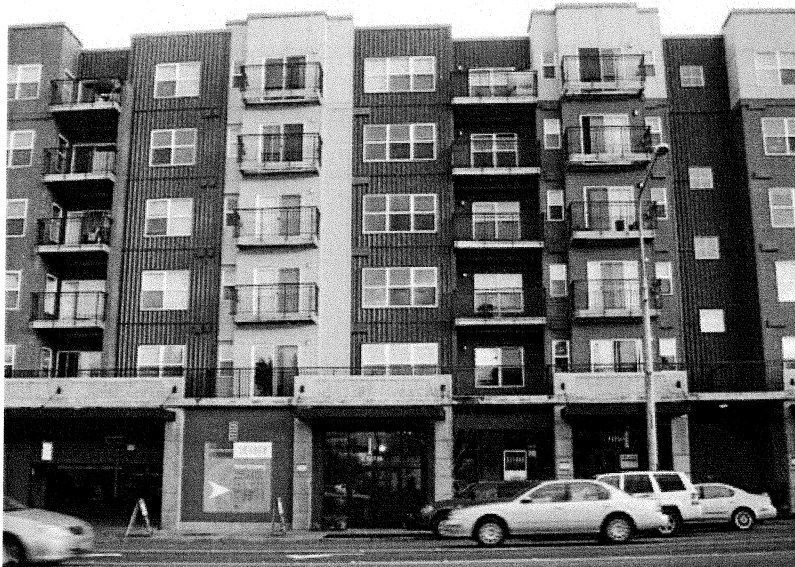
5 storey wood frame condos on a concrete podium in Seattle, Wash.
