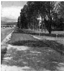
New pavement on Lochside Trail
