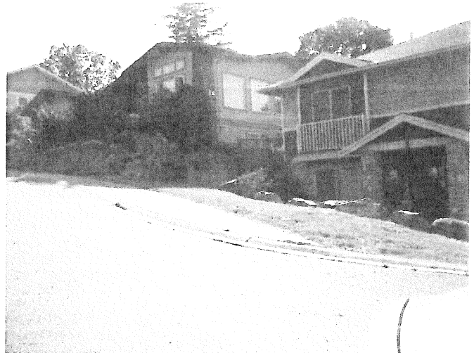
More boulders by roadside on a slope to prevent vehicles from sliding onto property
