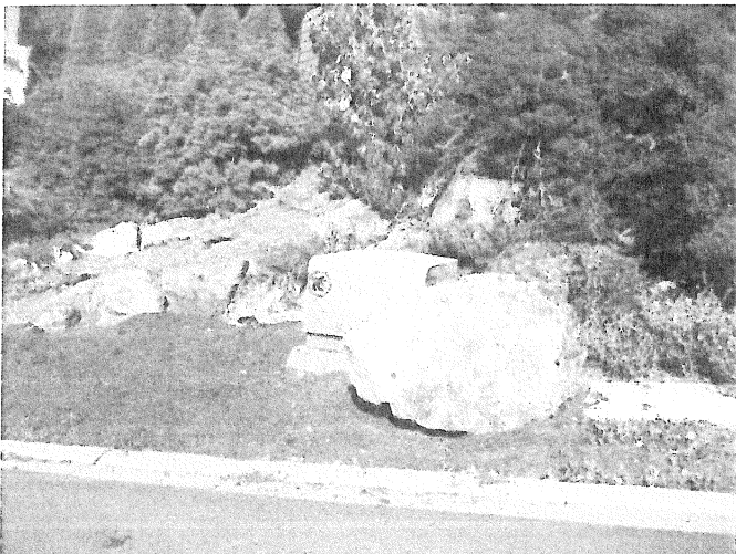
Boulder protecting electrical distributor box in area
