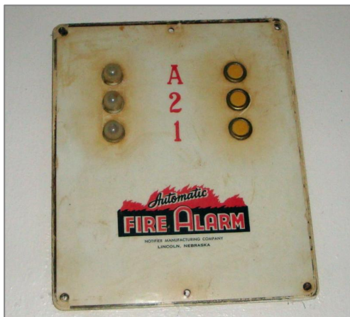
Outdated fire alarms pose a risk to life and property.
