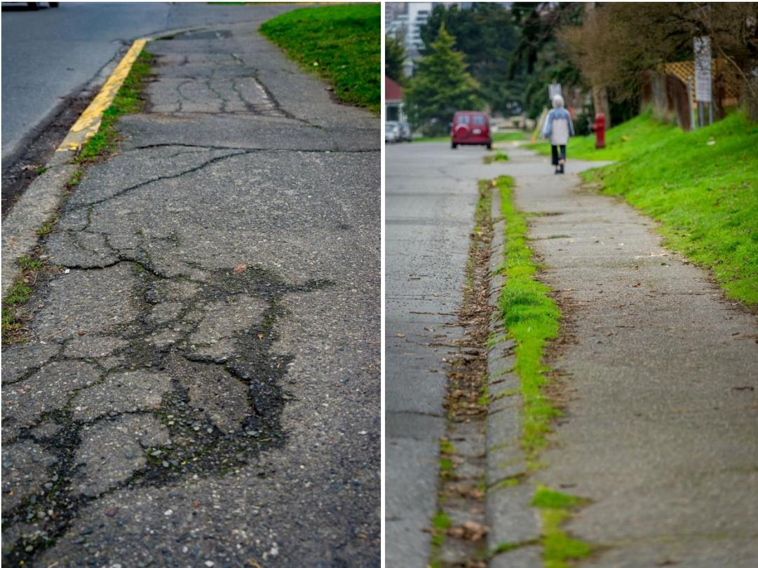
Examples of poor sidewalk condition on Lyall Street with cracking concrete sidewalk (left) and debris / uplift (right).
