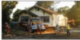
A crew prepares a Victoria home to be trailered and moved onto a barge. (Courtesy Ryan Goodman)
