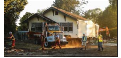
A crew prepares a Victoria home to be trilledered and moved onto a barge. (Courtesy Ryan Goodman)
