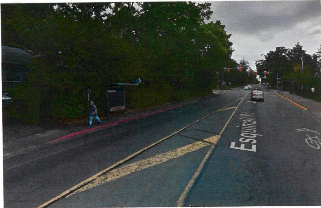
Figure 8: Existing Transit Stop on the Frontage
