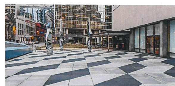
CONCRETE SLAB WITH GEOMETRIC CUT LINES
