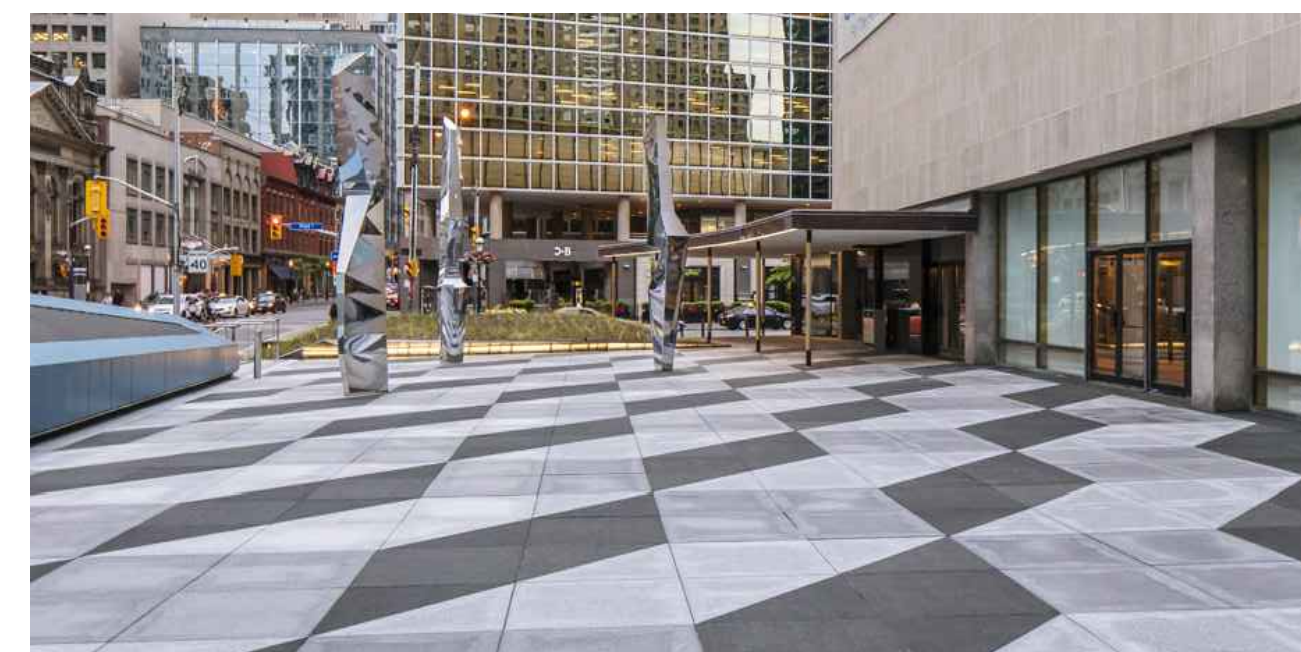
CONCRETE SLAB WITH GEOMETRIC CUT LINES
