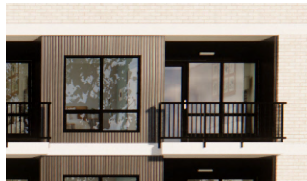
PREFINISHED ALUMINUM RAILING - RAILS
