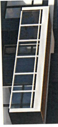
PREFINISHED ALUMINIUM RAILING - GLAZED PANELS
