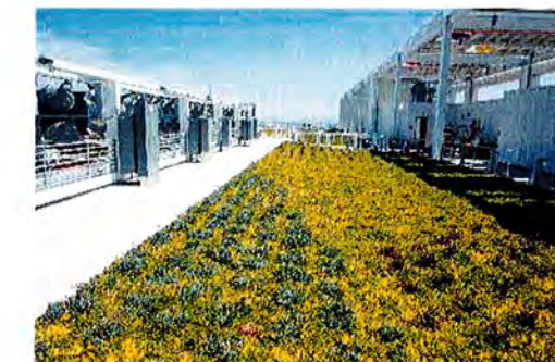
GREEN ROOF POTENTIAL ON LEVEL 2 ROOF
