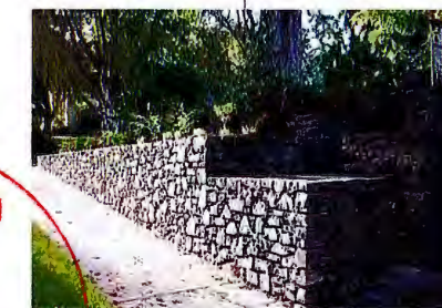
BLAST ROCK WALL
