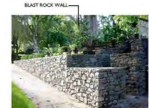
BLAST ROCK WALL
