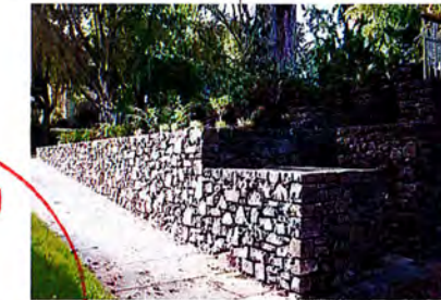
BLAST ROCK WALL
