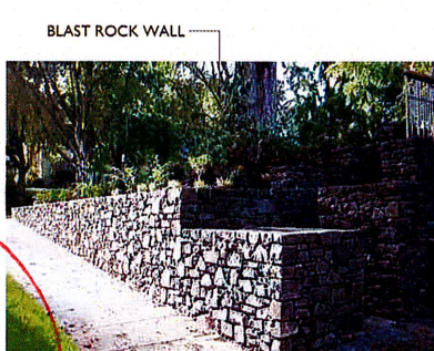
BLAST ROCK WALL
