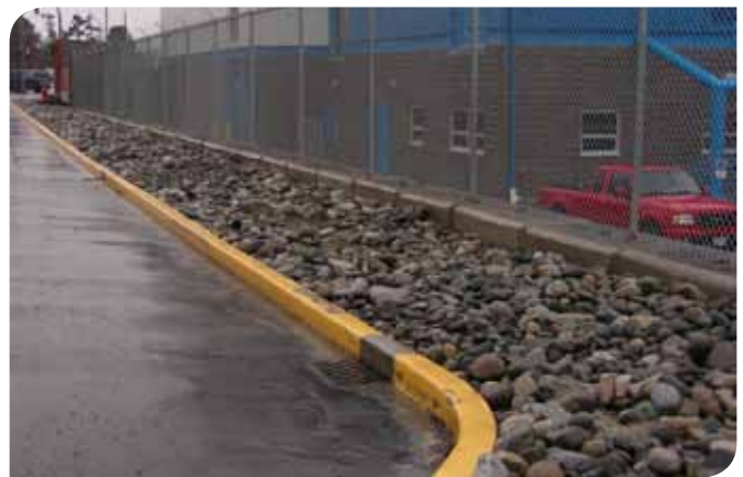
Boulevard and curb and gutter construction along Canteen Road.
