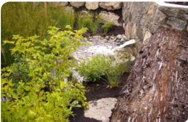
Storm water outfall into rain garden at Yarrow Place.
