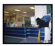
The Township recently built a glass window to protect individuals working at the front desk. However, the glass window ends right in the middle of the lower cut out section, which blocks the line of vision for someone seated in a wheelchair. Accessibility can be enhanced through widening the cut out section of the reception desk or extending the glass window so that there is no barrier.
