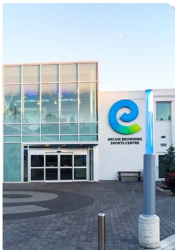
The Archie Browning Sports Centre benefitted from upgrades in 2018.
