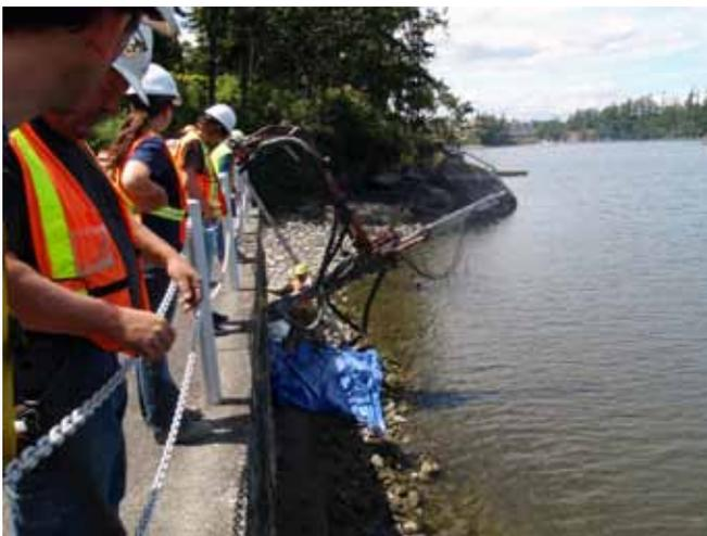
Drilling anchors into the Arm Street Seawall
