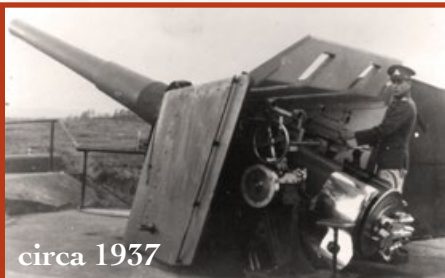
This was one of HMCS Rainbow's 6" breech-loading, quick-firing guns. They were placed at Fort Macaulay in 1924 after the ship (Canada's first navy vessel) was scrapped.
