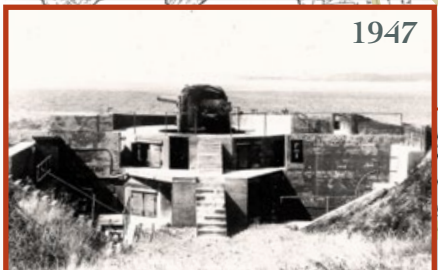
Six-inch Mk VII Breech-loading gun on the right emplacement.
