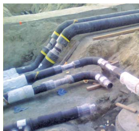
Laying of insulated district energy pipes for the South East False Creek Neighbourhood Energy Utility. The pipes will transmit water, warmed by heat recovered from wastewater, to heat the neighbourhood. Source: Community Energy Association
