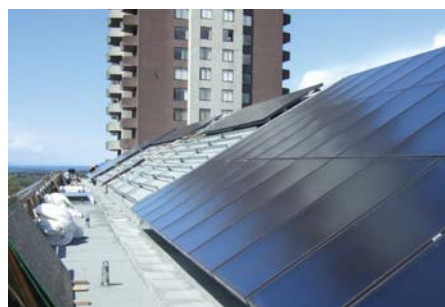
Solar hot water panels under construction on the roof of the City of North Vancouver public library.
