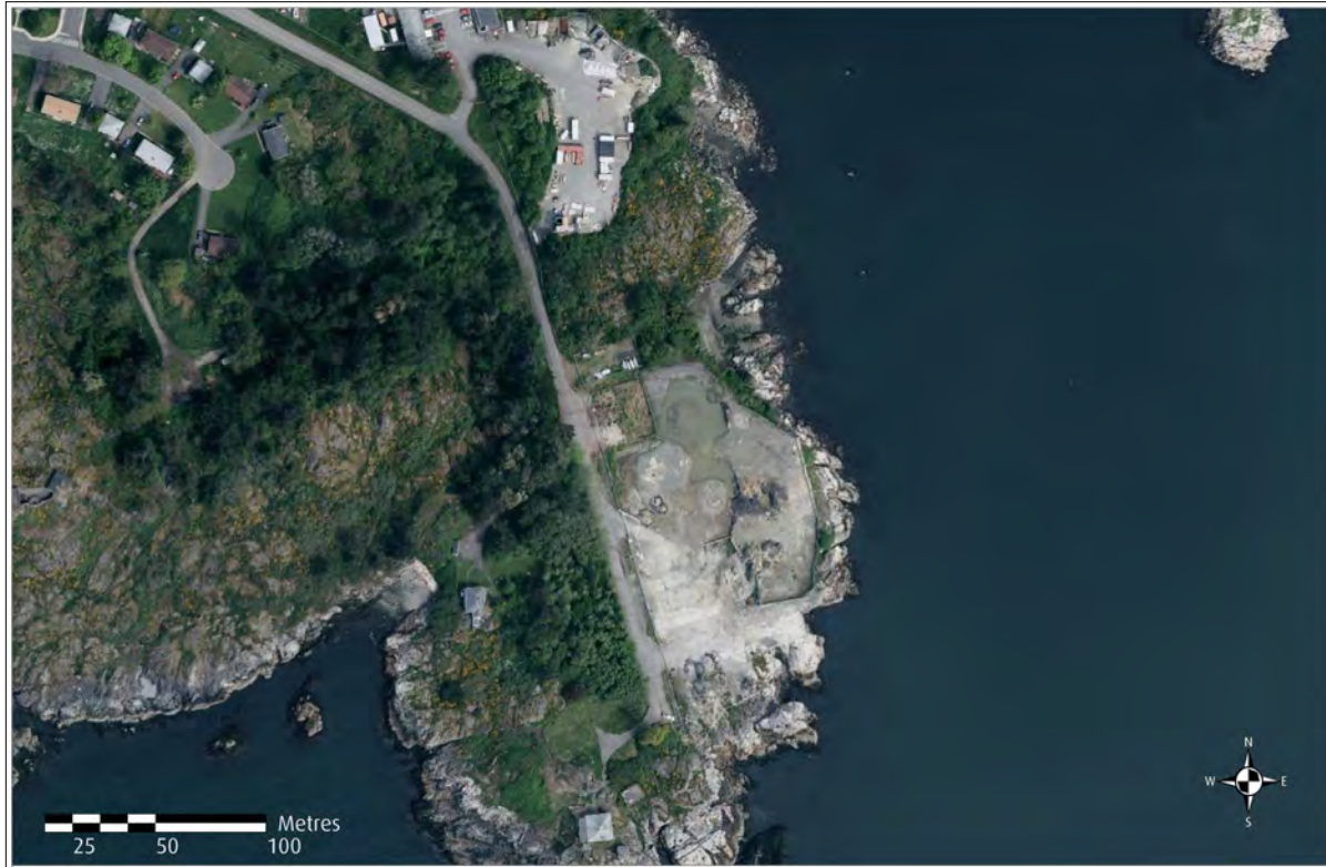
Figure 4: McLoughlin Point Current Conditions
