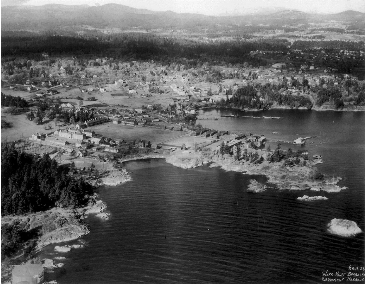
Work Point Barracks [Esquimalt Archives]
