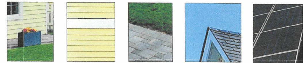
HARDIE SIDING & WHITE WINDOW TRIM (TO MATCH EXISTING) HARDIE SIDING & WHITE TRIM BOARDS (TO MATCH EXISTING) DADU PATIO (TO MATCH EXISTING) ROOFING MATERIAL (TO MATCH EXISTING) SOLAR PANEL
