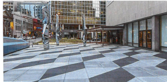
CONCRETE SLAB WITH GEOMETRIC CUT LINES
