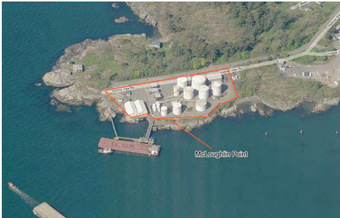
Figure 5-7 McLoughlin Point site before fuel tank decommissioning in 2008
