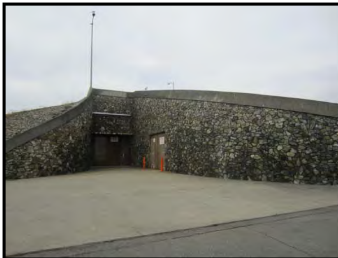
SOUTH ELEVATION OF CLOVER POINT PLANT
