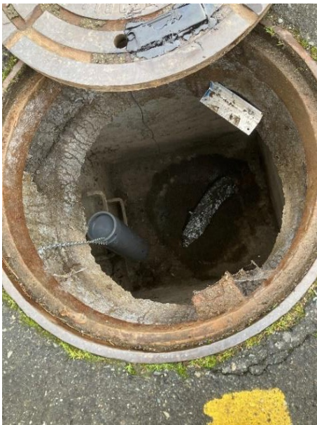
Figure 7-1: Ultrasonic Level Logger Setup
