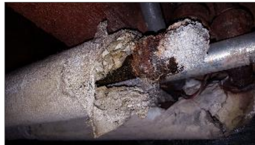
Aircell insulation in poor condition, Location 7
