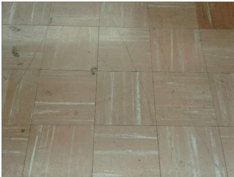
9x9 VFT Red/pink with white streak, Location 6 (S009A-C, Asbestos containing)
