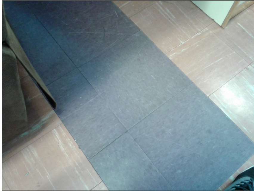
12x12 Purple VFT, Location 6 (S0012A-C, non-containing)
