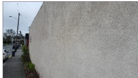
Texture finish on the exterior, Location 10
