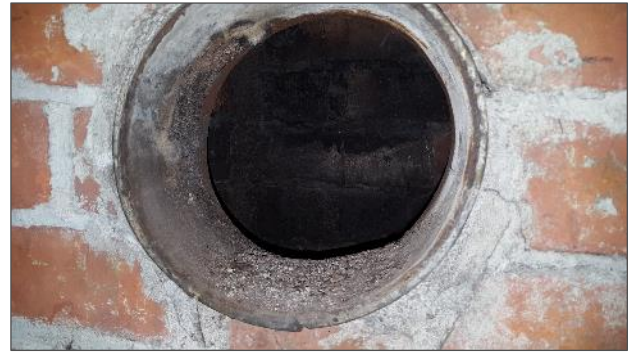
Former chimney mortar and debris, Location 2
