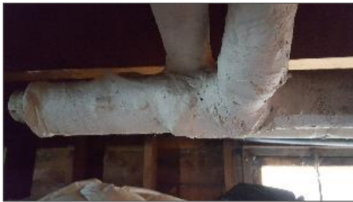
Parging cement insulation, Location 7
