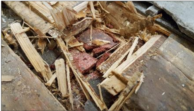
Asbestos-containing VFT below wood subfloor in #1239, Location 2
