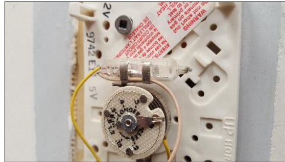
Mercury in thermostat in Location 1.
