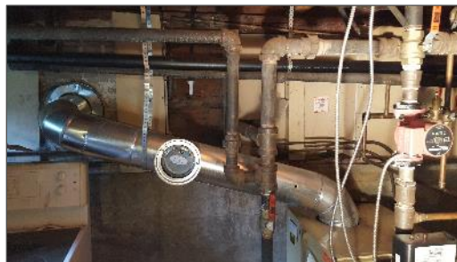
Bell & Spigot Piping, Location 7
