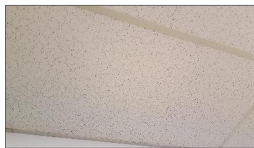
Lay in ceiling tiles (2010), Location 1
