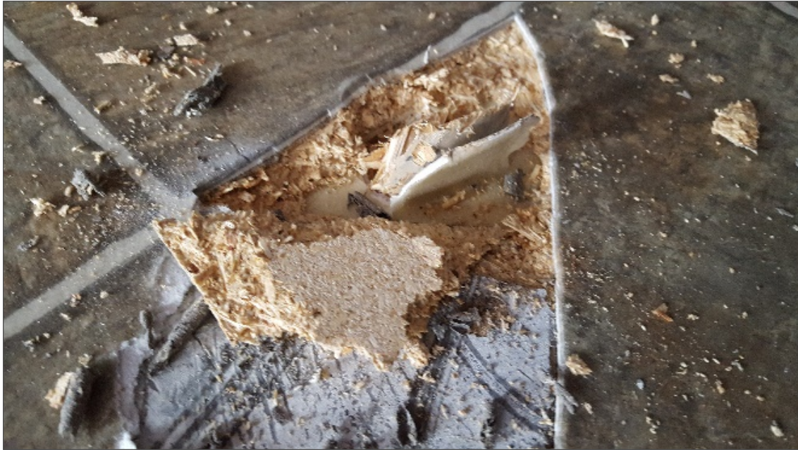
Unidentified white foam between wood layers, Location 8 (S0019, non-containing)
