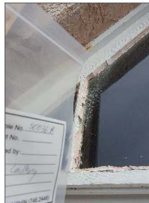
White window caulking, Location 10
