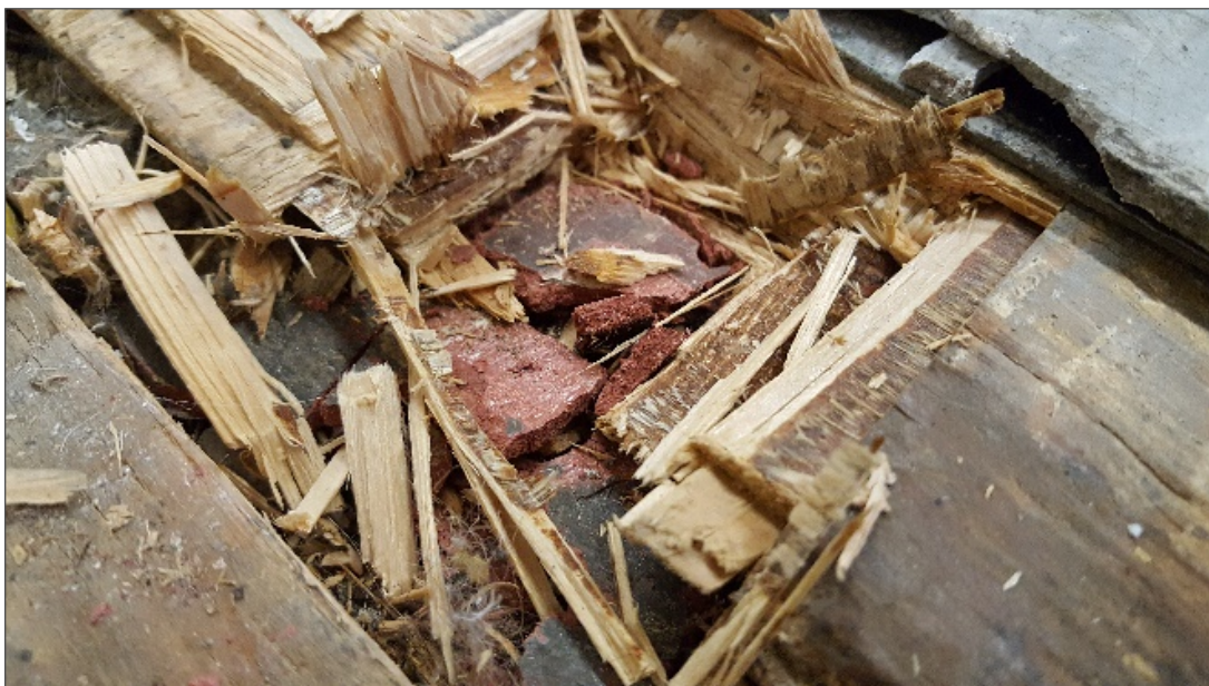
Unidentifiable VFT & Red VFT, Location 2 (S006, S007, Asbestos containing)
