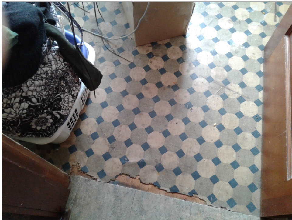
VSF Brown/black checker, Location 9 (S0030, Asbestos containing)
