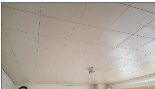
White glue on ceiling tiles in 2 nd floor residential, Location 9
