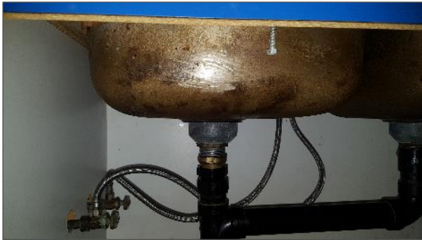
Black Mastic under the sink, Location 8
