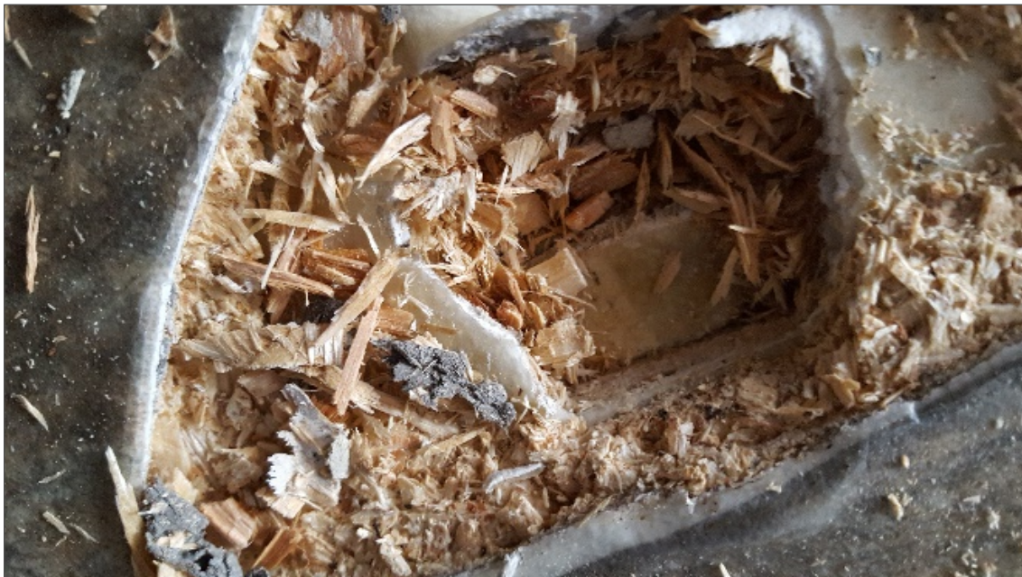
VSF with backing paper below layers of wood, Location 8 (S0020, Asbestos containing)
