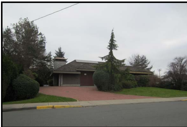
LOOKING SOUTH TO PUMP STATION BUILDING ON CURRIE ROAD
