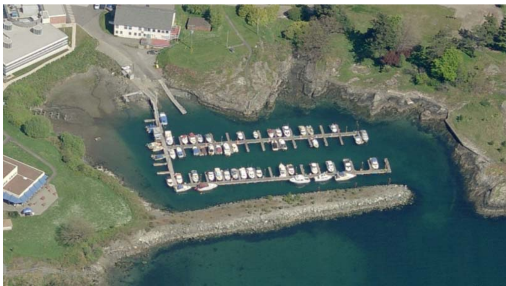
Figure 5-6 CFB Esquimalt marina, north of the McLoughlin Point site
