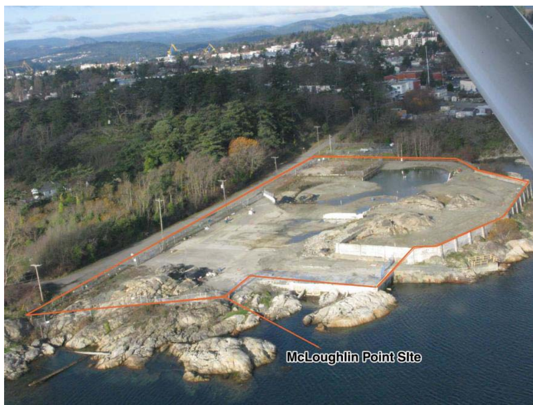
Figure 5-1 McLoughlin Point site from south
