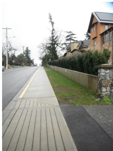
Figure 2 - Boulevard with adjoining sidewalk
