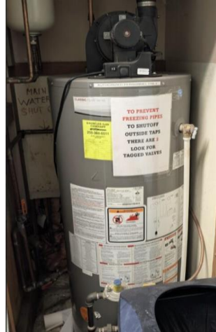
Figure 3-4 Domestic Hot Water System
