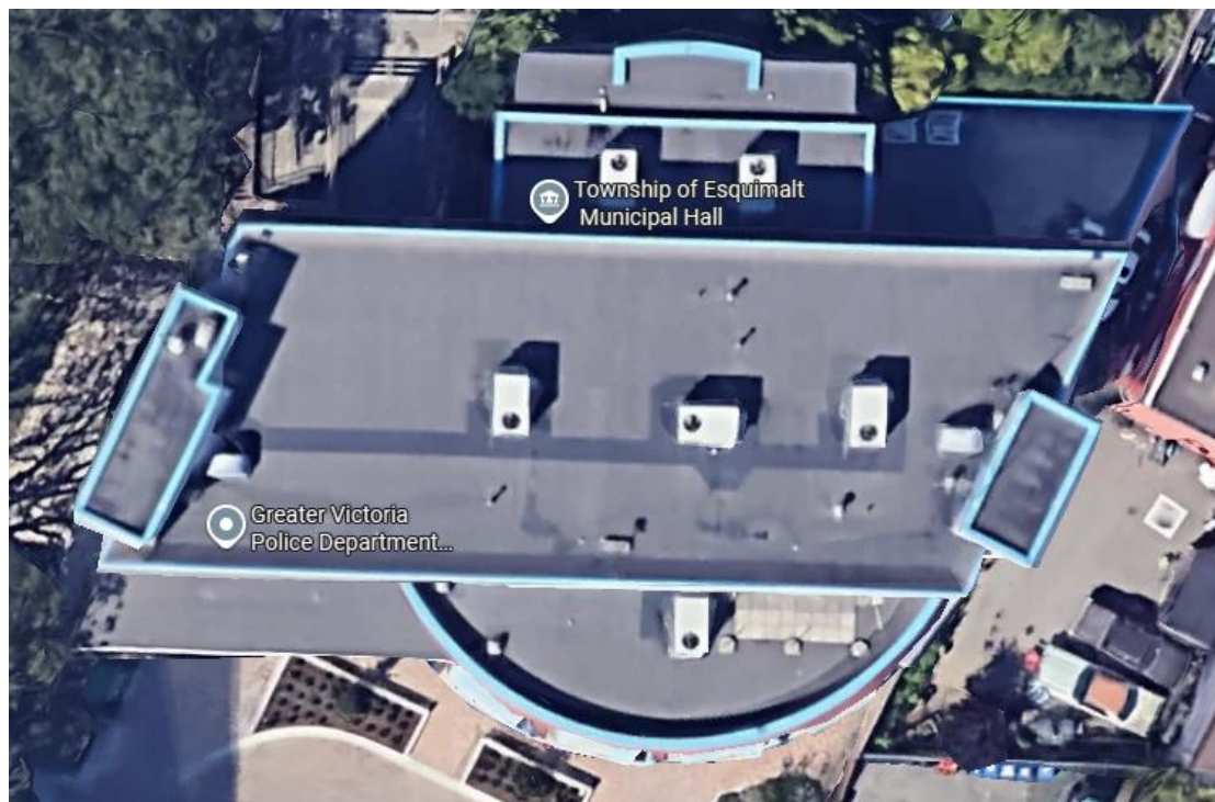
Figure 3-1. Aerial view of the Municipal Hall
