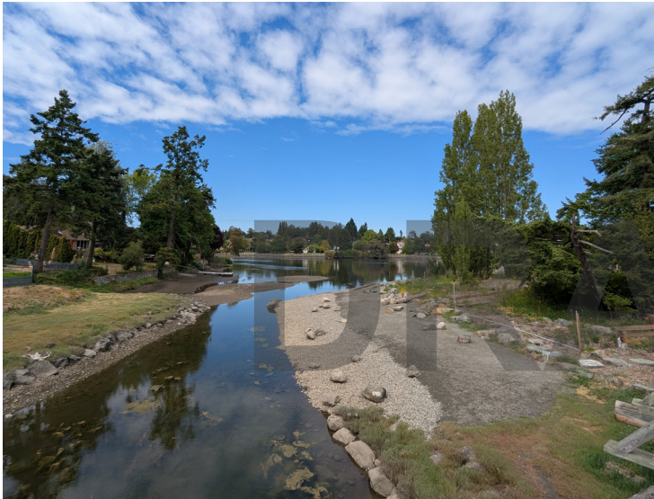
Shoreline rehabilitation in progress.
