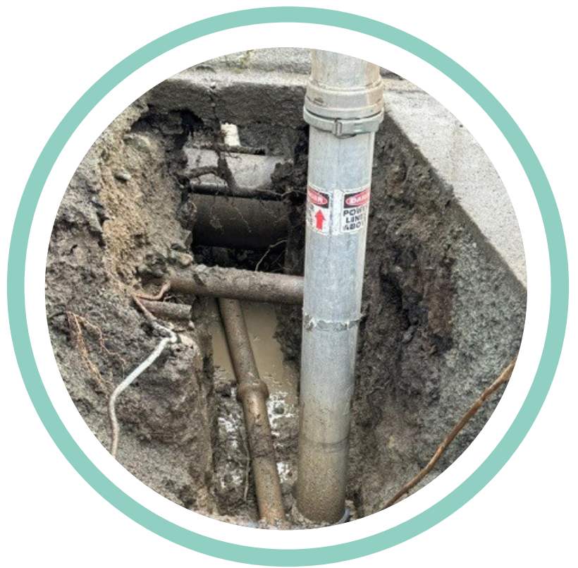
Public Works exposing utilities to repair a sewer.
