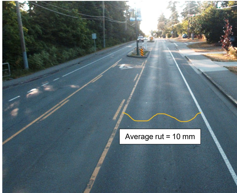
Figure 6: Segment on Craigflower Road Showing Low-Severity Rutting
