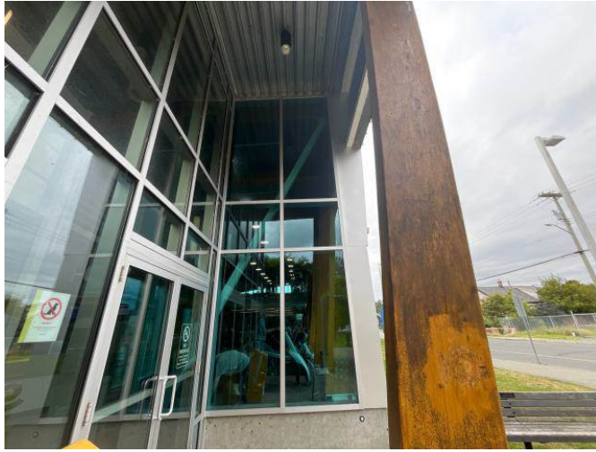
Photo #10: Entrance Window-Wall
