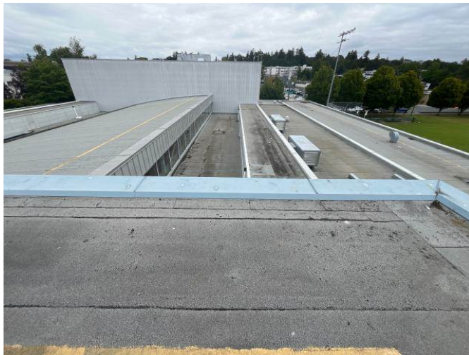
Photo #9: Flat Roofing - General Condition (3)
