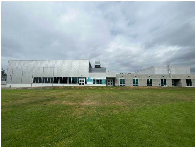
Photo #2: East Elevation
