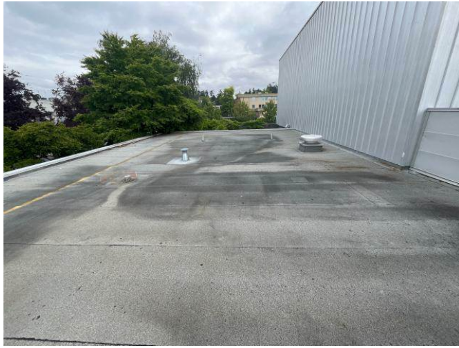
Photo #7: Flat Roofing - General Condition
