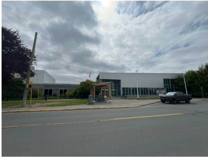
Photo #4: West Elevation
