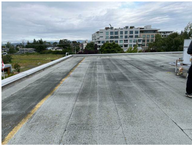
Photo #8: Flat Roofing - General Condition (2)
