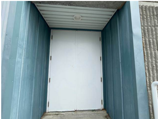
Photo #12: Service Door - Typical
