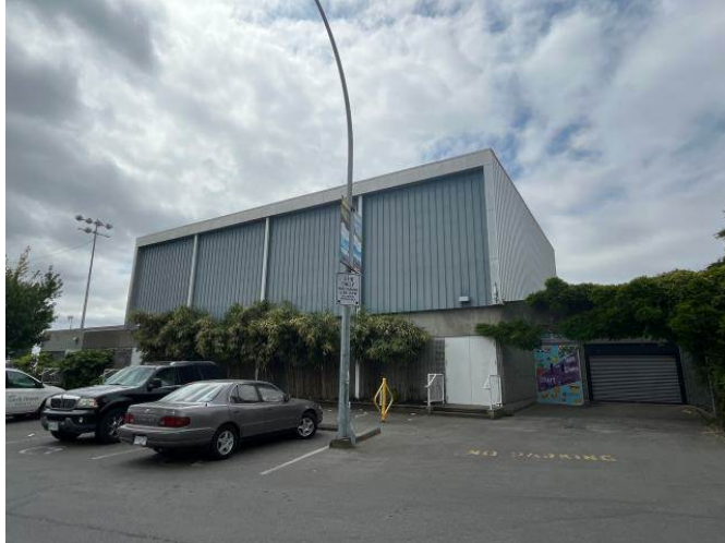
Photo #1: North Elevation
