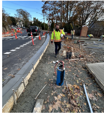
Work along Esquimalt Road.
