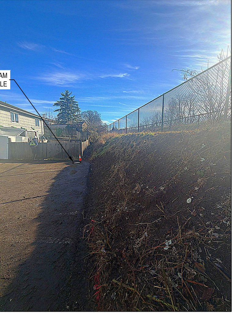
PHOTO #2 855 ADMIRALS RD FENCE LINE Scale N.T.S.
