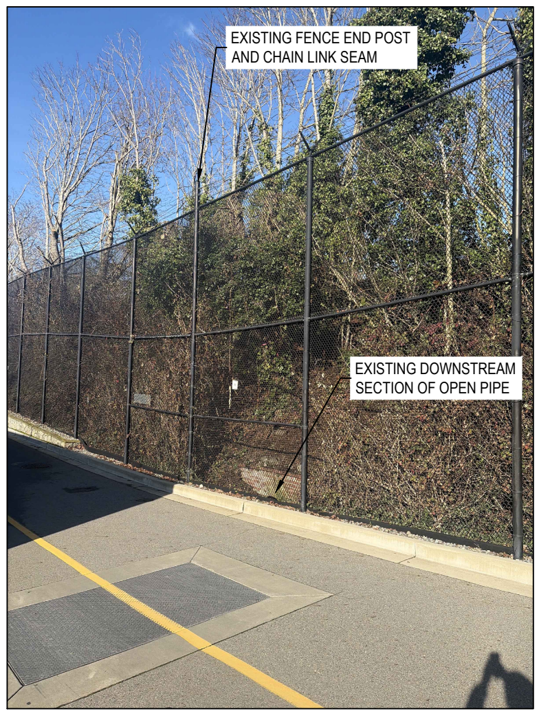
PHOTO #1 PSPC FENCE LINE Scale N.T.S.
